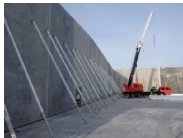
Figure 20.23 – Bracing Panel while Construction Progresses
