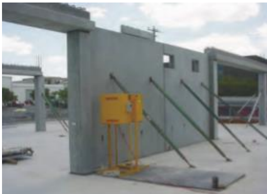
Figure 20.13 – Internal Precast Wall Panels – loadbearing walls to support precast flooring
