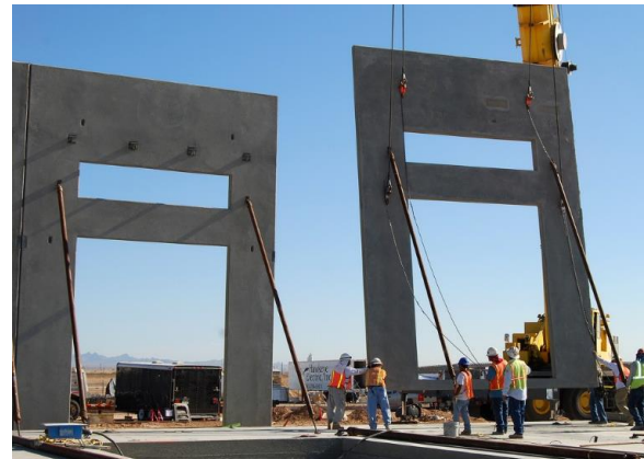
Figure 20.22 – Bracing of Precast Panel – Braces fixed into Slab Floor and Panel 20.2
